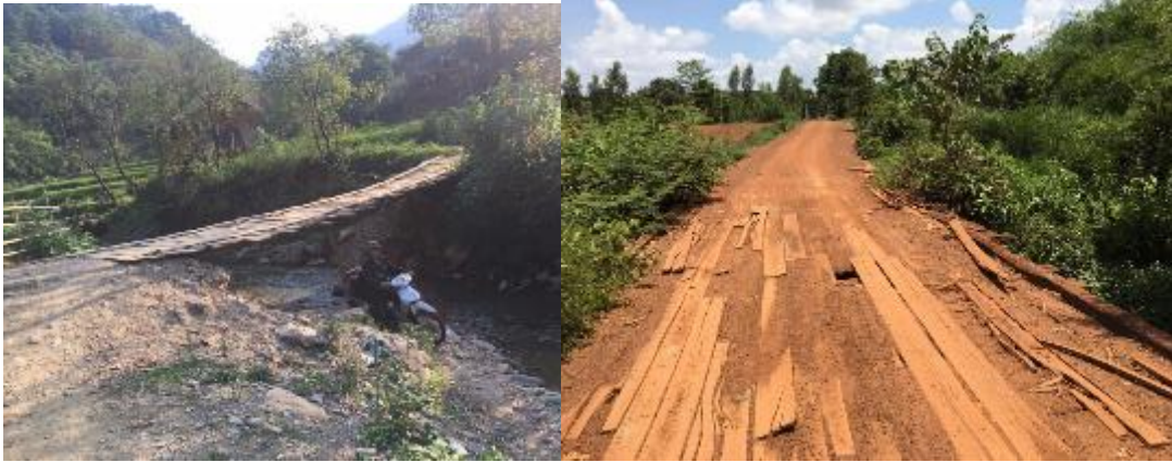
Many bridges in Vietnam are temporarily built and unsafe
